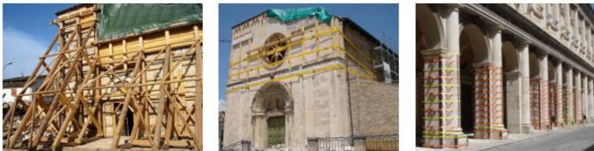
Figure 14 - Temporary consolidation procedures [9]
