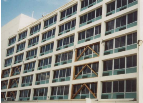
Figure 15 – Shoring used in Northridge [11]
