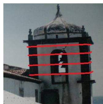
Figure 19 - Solution wrap the tower
