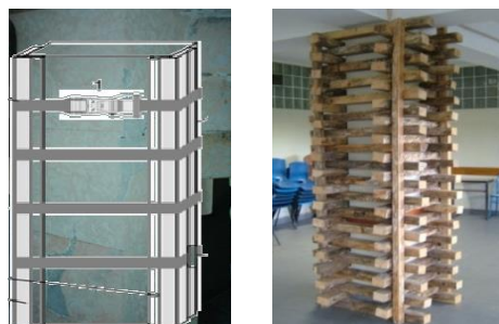
Figure 18 - Solutions of shoring and B-pillar reinforcement
