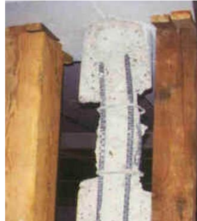
Figure 15 – Shoring used in Northridge [11]
